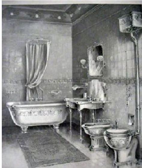
The bathroom George had arranged to be installed.
